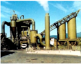
Bridgewater asphalt plant—high capacity with hot storage facilities
