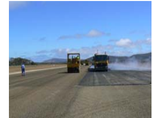
Spray sealing—Flinders Island Airport
