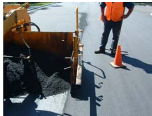
Laying asphalt through a paver
